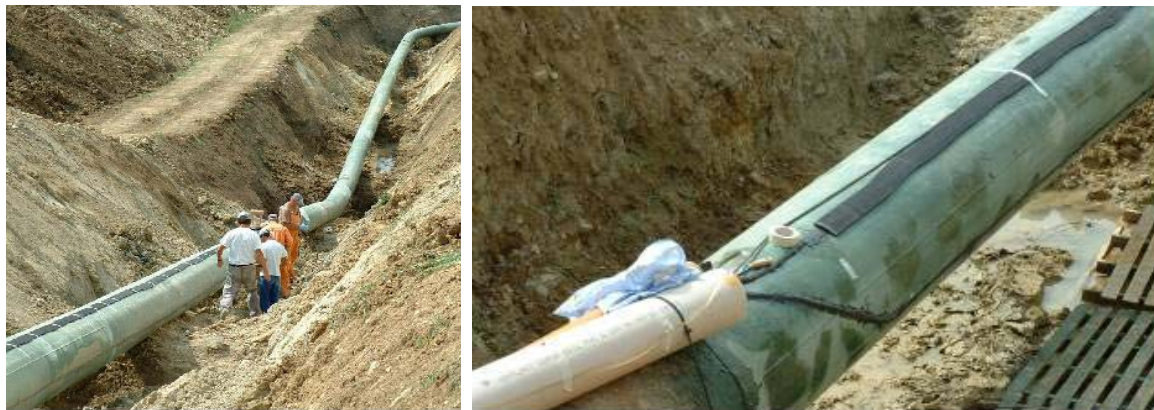
Figure 3: Example of SMARTape integration on a pipeline for strain monitoring
